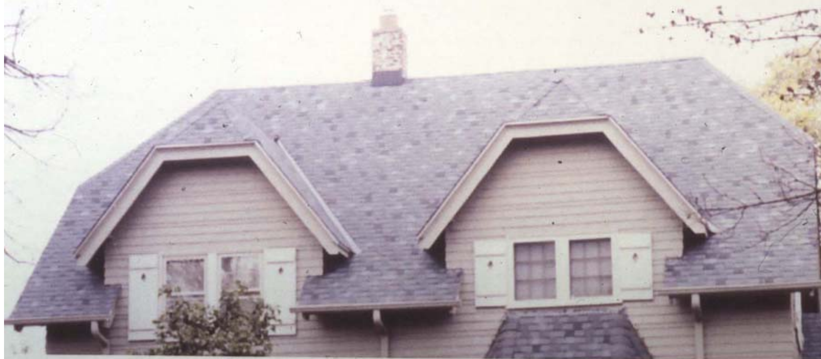
Completed roof project
