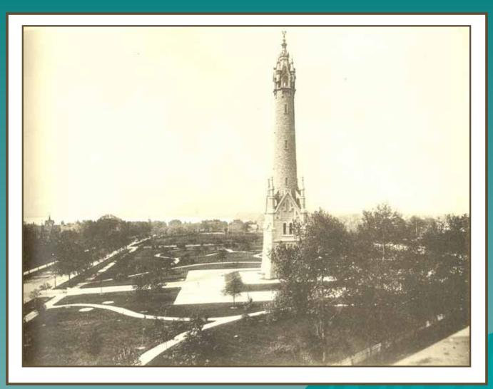
Built in 1873, out of Wauwatosa-cut limestone, the North Point Water Tower soon became an object of pride in Milwaukee.
